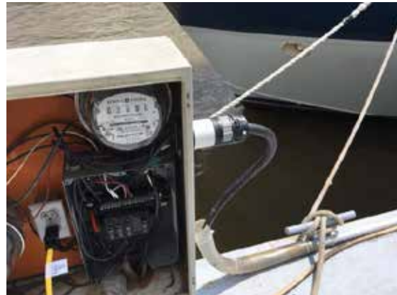
New plug and rewired dock box
